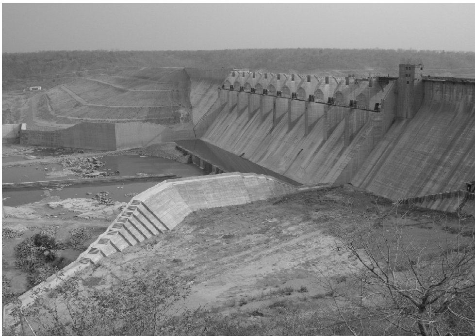
Fig. 1 : Shows MDP site in Madikheda village in the Sindh River
